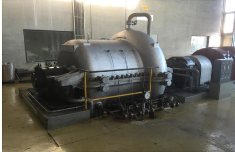
and the compressor housing. This results in all kinds of damage, such as deformation of the internal body parts, resulting in leaks and steam reflow. These phenomena badly affect the compressor's uptime and efficiency and could even lead to complete standstill. In that case the factory cannot dry any more salt since this installation is crucial to the production process.
